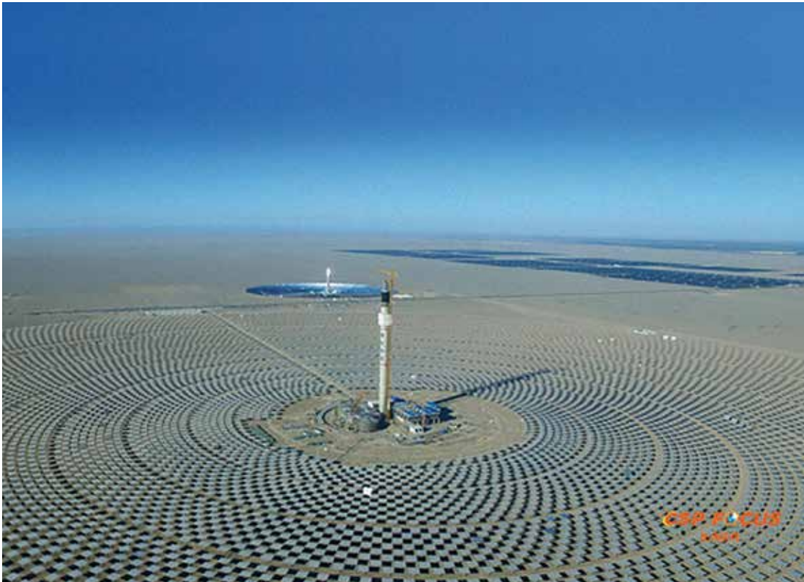
IMAGE CREDIT: PROTERMOSOLAR, China Shouhang Dunhuang 100 MW molten salt Solar Tower Concentrated Solar Power Plant
